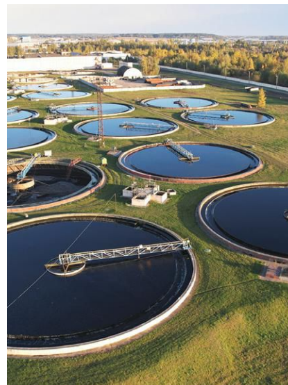
IMAGE 5: Wastewater treatment facility
